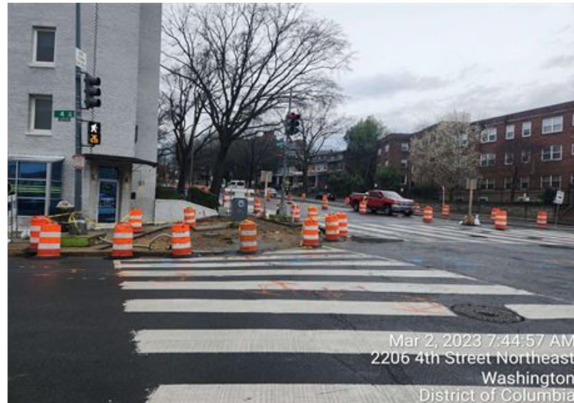
4 th Street Restoration
