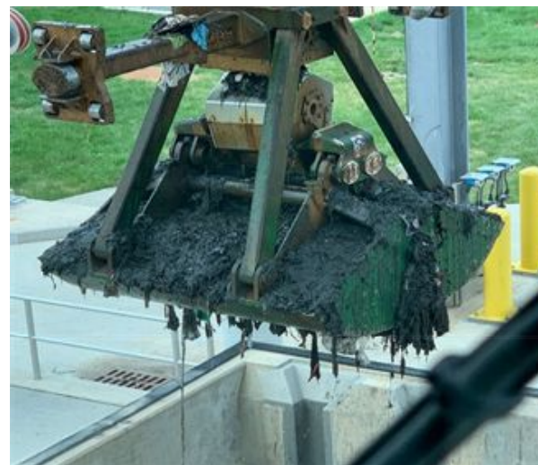
Trash, Debris and Solids Removal from Screening Shaft at Tunnel Dewatering Pumping Station
