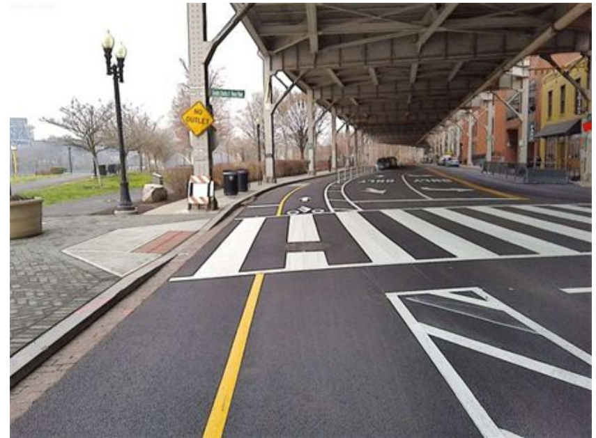
Finished Pavement at the Intersection of Wisconsin Avenue and K Street
