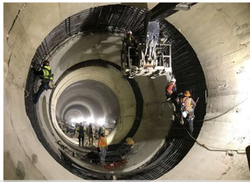
FLA Adit Repair
