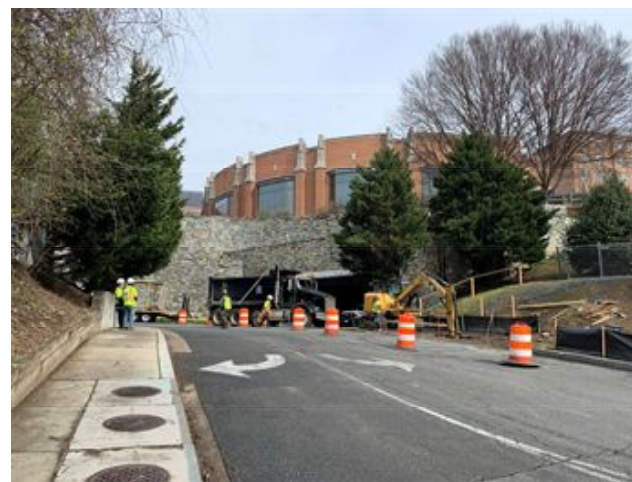
Installing CSO-029 Electrical Manhole at Entrance to Georgetown University
