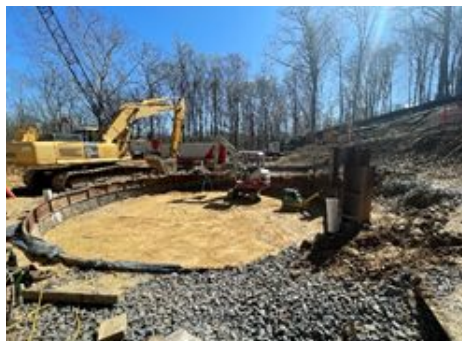
Completed backfill of the slip line shaft
