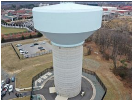
St. Elizabeth Elevated Water Tank
