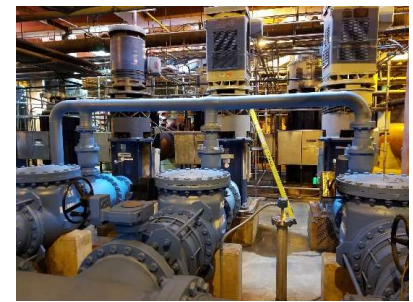
Reclaimed Final Effluent Pump Station Upgrades
