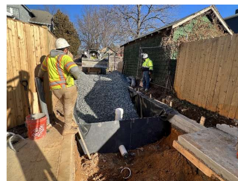
Alley Permeable Pavement
