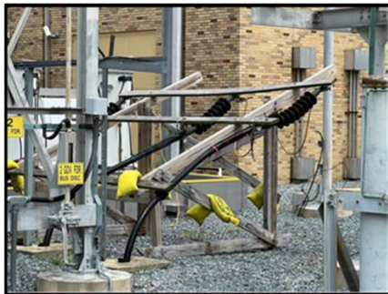
NRL Feeder Upgrades
