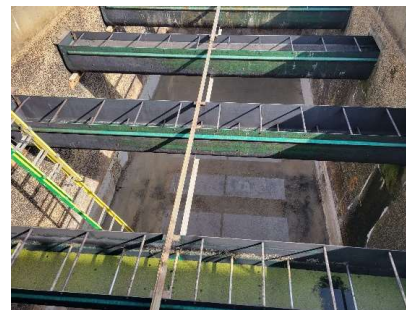
Interim Filter Rebuild Project
