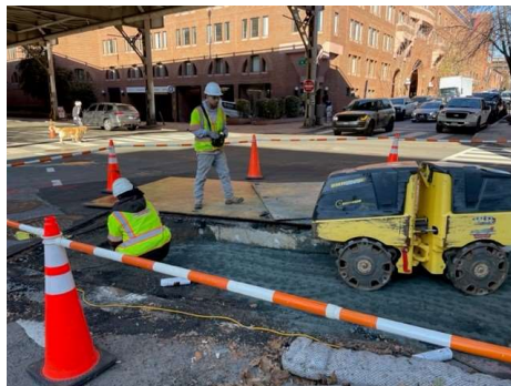
Restoration at CSO 024
