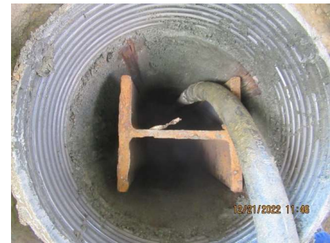
Pile #4 at Str 44
