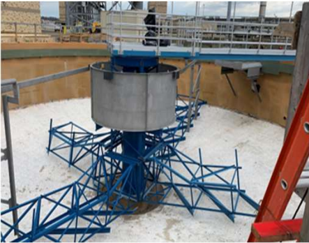
Gravity Thickener Upgrades GT-1 through GT-10
