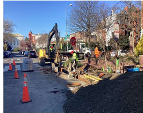
SDWMR 12C: Water Service Replacement at Tuckerman St, NW
