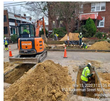
SDWMR 12C: Water Service Replacement at Tuckerman St, NW
