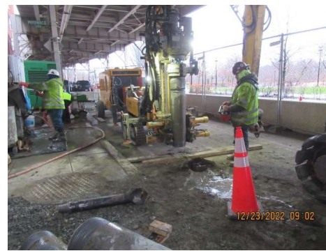
Str 44 Work at Wisconsin Ave
