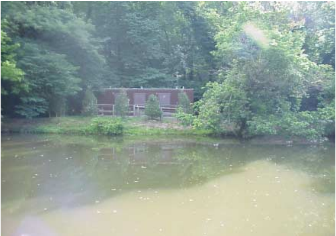
Figure 10d.1: Existing Summer View 10d at Site 1995 from C&O Canal Towpath (leaves-on)
