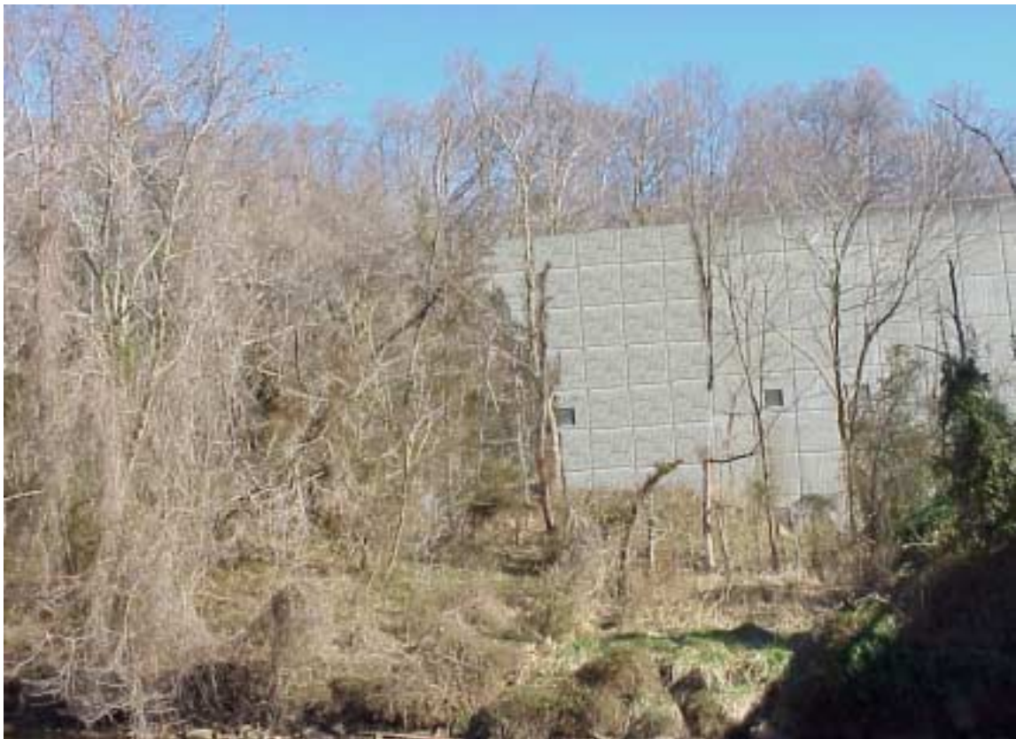
Figure 9d.4: Building Rendering at Site 4 from Winter Viewing Direction 9d (leaves-off) (Building rendering is provided as an example, which is subject to final approval by the NPS and SHPOs)
