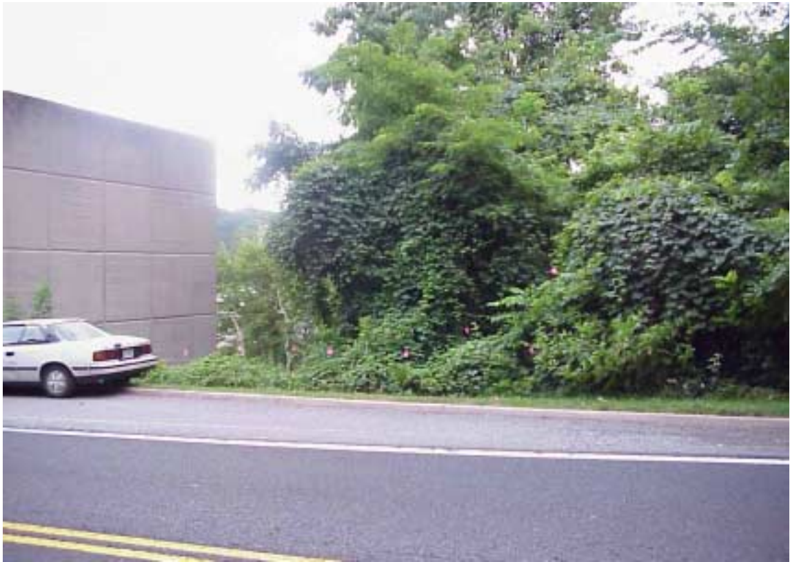
Figure 9c.1: Existing Summer View 9c at Site 4 from Clara Barton Parkway (leaves-on)
