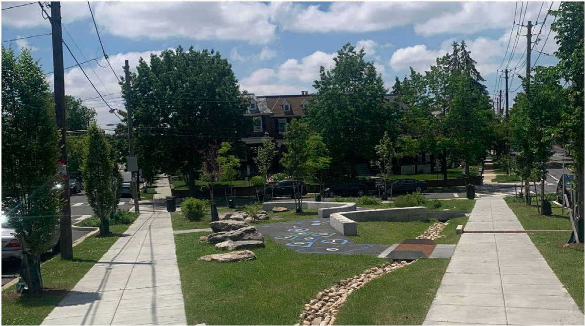
Figure 2-4. Typical GI Park (photo)
