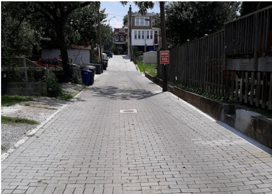
Figure 2-8. Typical Green Alley Partnership Installation (photo)
