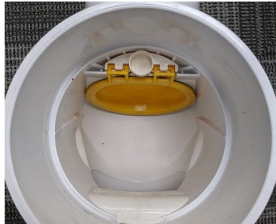
Figure 2-15. Flow Restriction Device – Flapper Style
