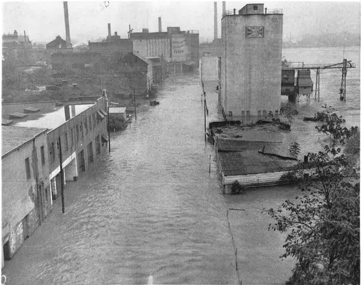
Water St. looking east during the October 1942 flood. The cement silos for the Lone Star Cement company are slightly east of 34 th and Water streets.
