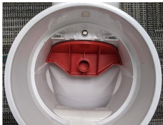
Figure 2-18. Flow Restriction Device - Straight Fit Gate
