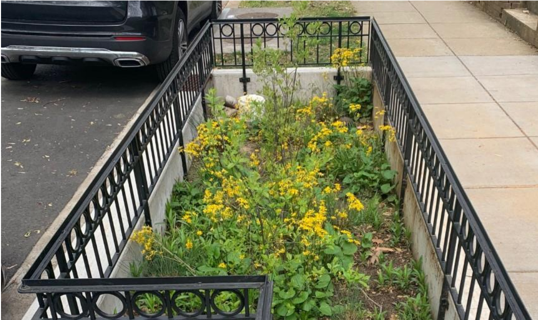
Figure 2-7. Typical Bioretention in Potomac Sewershed (photo)
