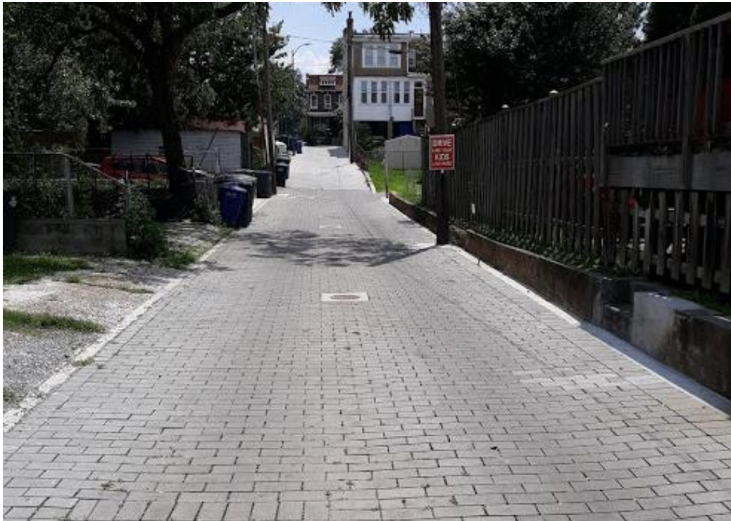
Figure 2-9. Typical Green Alley Partnership Installation (photo)
