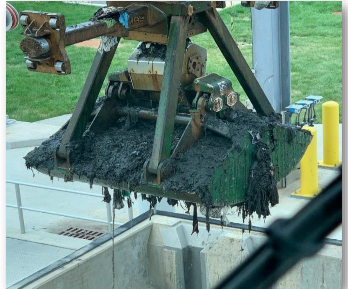
Trash, Debris and Solids Removed at Blue Plains from Anacostia Tunnel System
