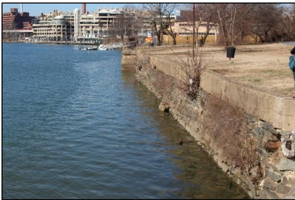
Figure 3-7: View of historic seawall topped by contemporary seawall
