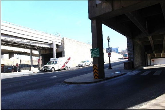
Figure 3-20: Eastern edge of proposed site, looking east; this portion of the roadways are not within the site
