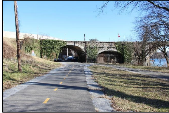
Figure 3-27: Western edge of proposed site, looking east at Aqueduct Abutment and Pier
