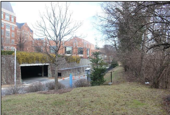
Figure 3-30: East corner of proposed site, looking east
