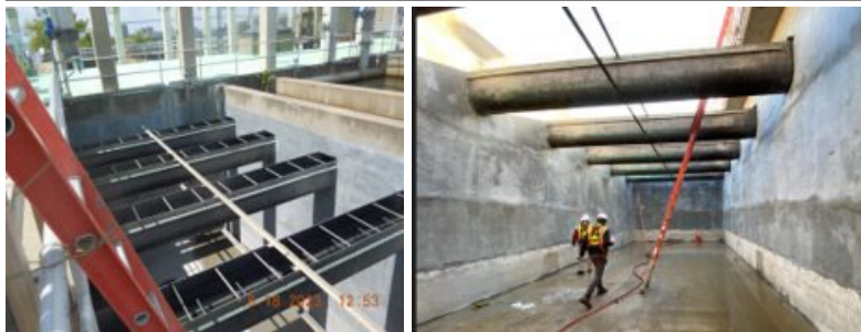
Filter Underdrain Replacement
