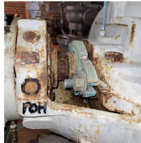
Figure C.25: Pump Packing, Typical
