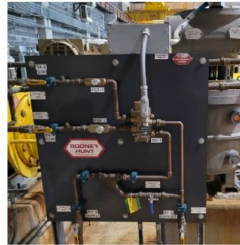
Figure C.13: Cone Valve – Typical Control Panel
