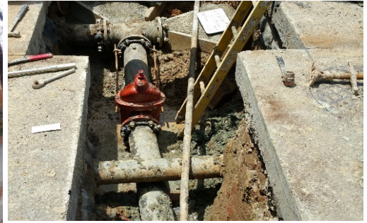
Small Diameter Water Main Florida Avenue & Sherman Avenue NW
