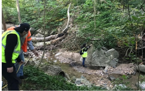
Rock Creek Stem Sewers (Condition Assessment)
