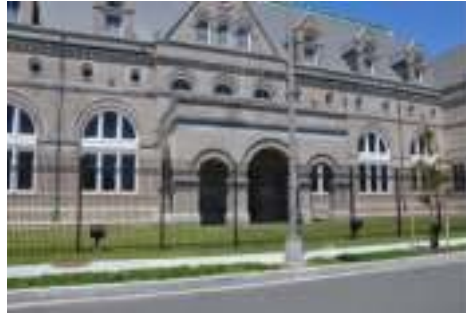
Bryant Street Pump Station
