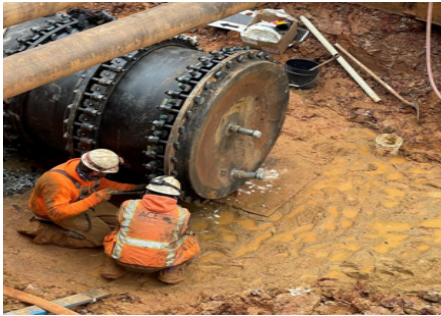
Soldier's Home Reservoir Upgrades
