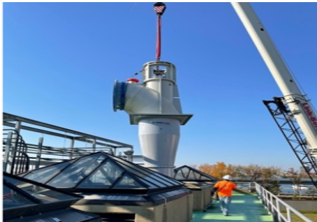
Blue Plains Filter Influent Pump Install
