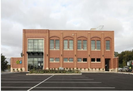
Non Process Facilities Sewer Building
