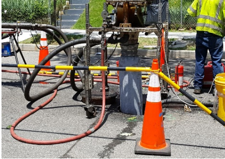
Sewer Rehab (Watts Branch)
