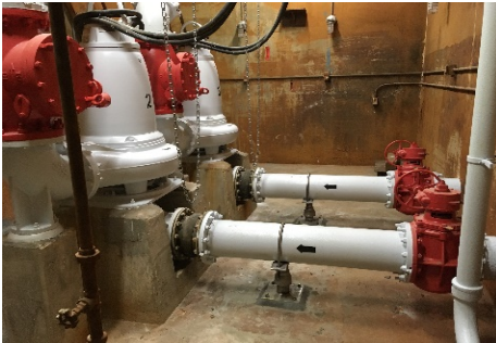
City Street Catch Basin
