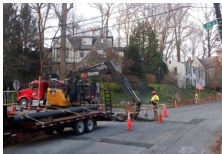
Small Diameter Water Main Rehab
