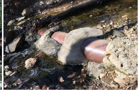
Sewer Rehab (Pinehurst Sewer)
