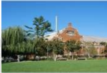
Main Pumping Station
