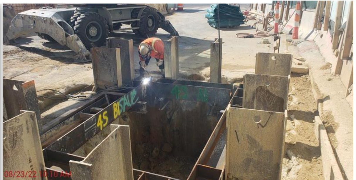
Ventilation Vault 2 Support of Excavation Installation
