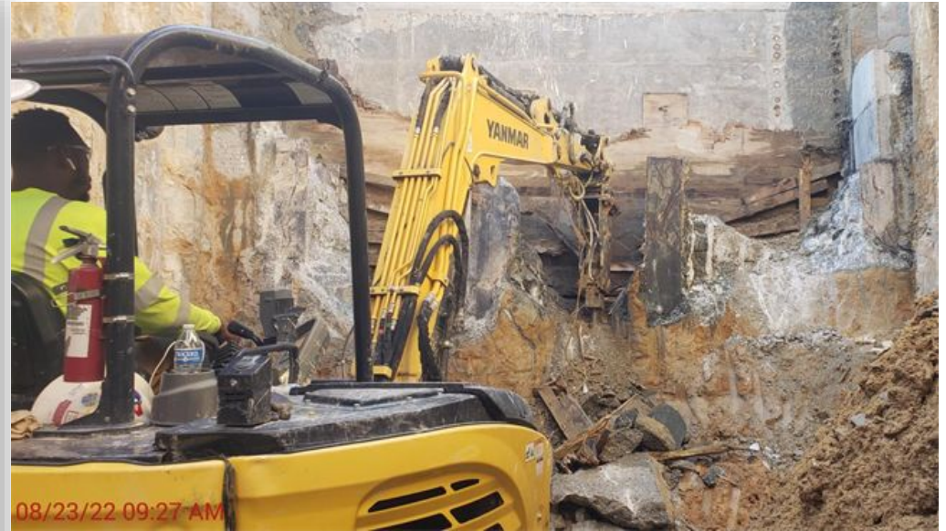
Approach Channel Excavation
