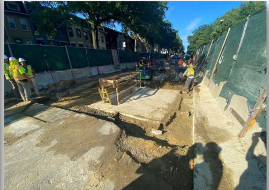
Construction Staging Area 2
