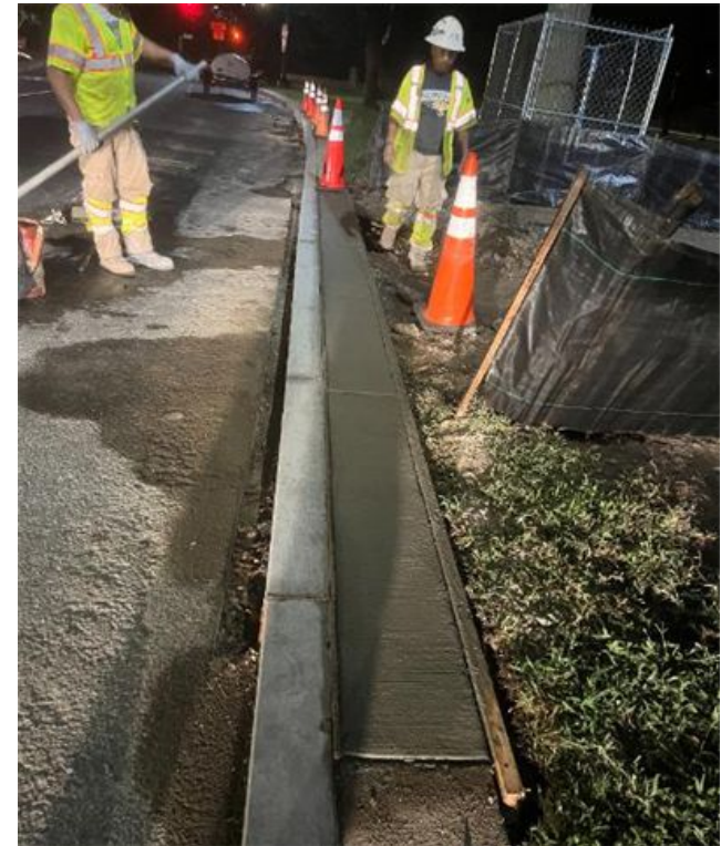
Final Restoration on Independence Avenue
