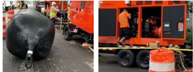
Contractor Pumps and Bypass Plug @1449 Florida Avenue, NW
