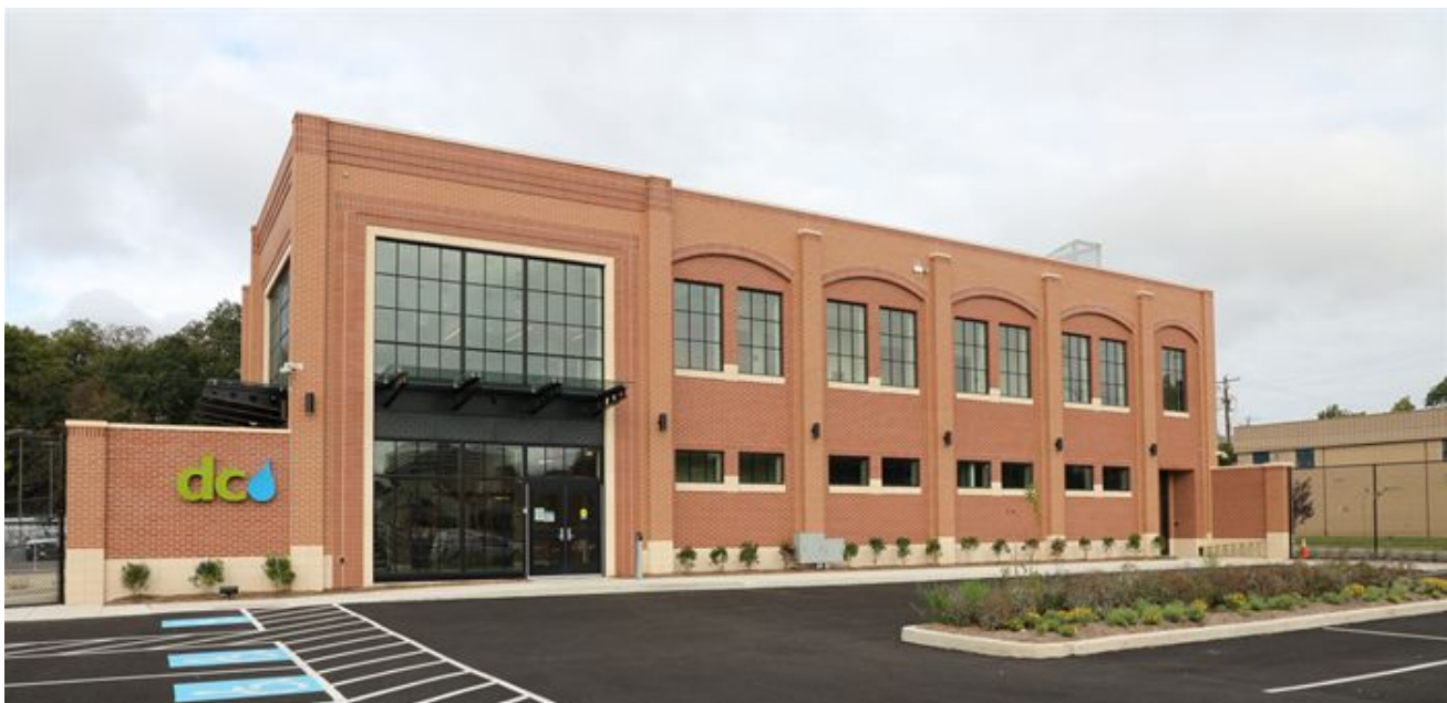
New Sewer Services Facility located on Ames Place, NE
