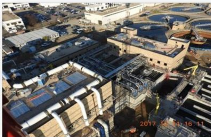
Figure 2. Wet Weather Treatment Facility Aerial View
