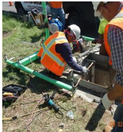
Kenilworth Ave. pump station upgrades
