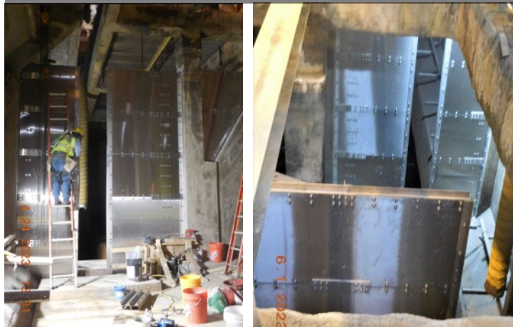
Grit Chamber Baffle Wall Project
