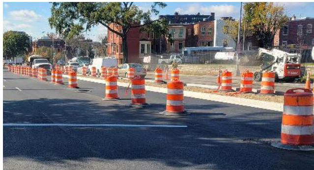
Florida Ave Restoration
