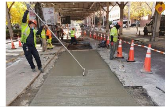
Road Restoration at CSO 024
