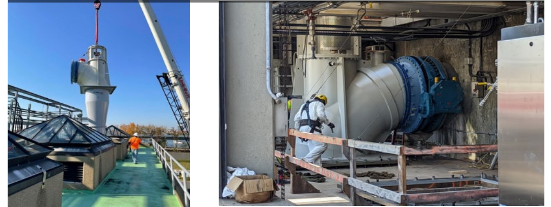
Filter Influent Pumps 1-10 Replacement Project
