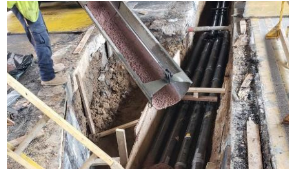
Duct Bank Work at CSO 024
