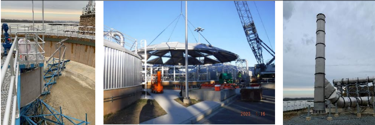
Gravity Thickener Upgrades GT-1 through GT-10
