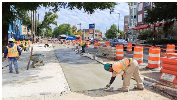
Rhode Island Ave Restoration
