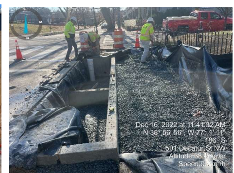
Planter Bioretention
