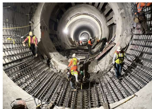
Liner at Florida Ave Adit
