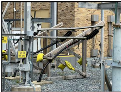
NRL Feeder Upgrades
