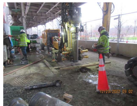
Str 44 Work at Wisconsin Ave
