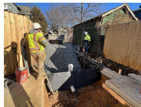
Alley Permeable Pavement
