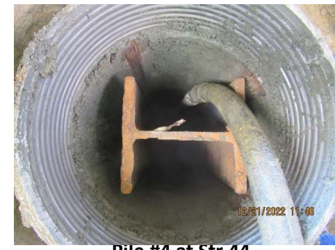
Pile #4 at Str 44
