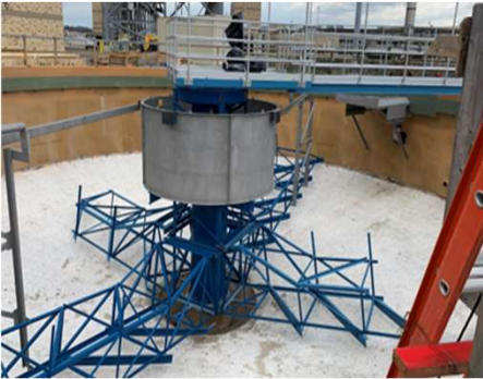
Gravity Thickener Upgrades GT-1 through GT-10
