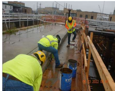
Process Basin Concrete Repairs
