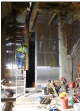
Grit Chamber Baffle Wall Project
