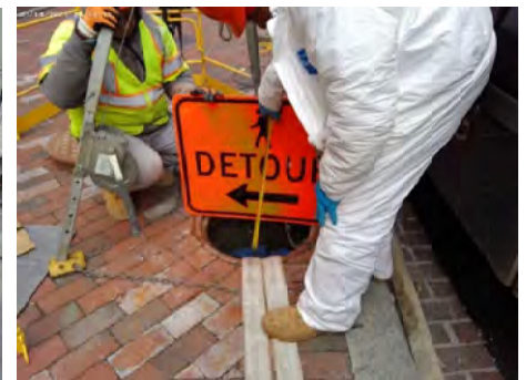
31 st Street – Manhole Testing
