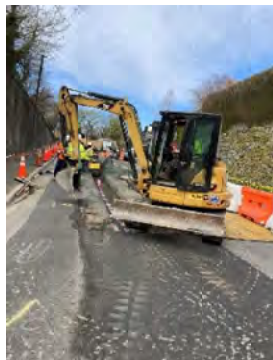
Backfilling Duct Bank at CSO 029
