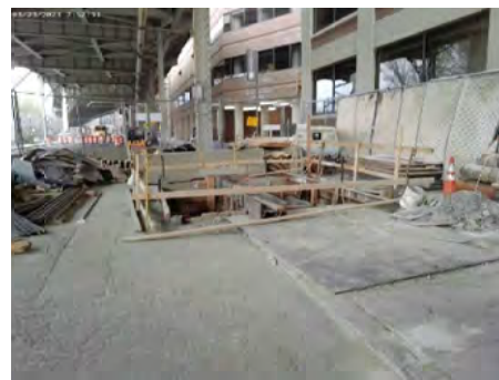
Str 44 Work at Wisconsin Ave
