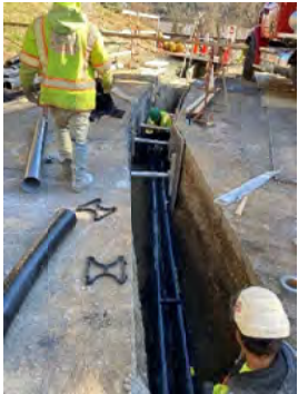
Installing Duct Bank at CSO 029
