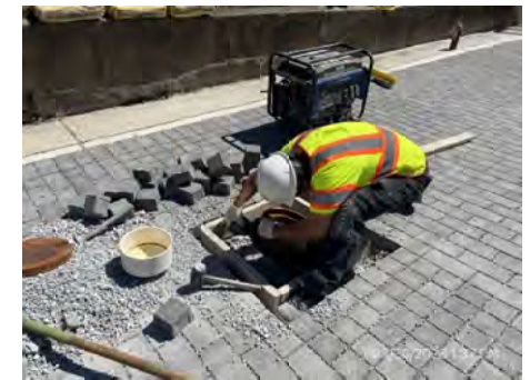
Alley Permeable Pavement (APP-66-08)
