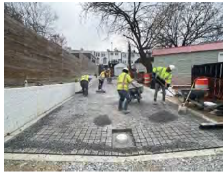
Alley Permeable Pavement (APP-51-05)
