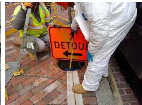
31 st Street – Manhole Testing
