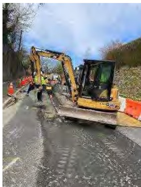
Backfilling Duct Bank at CSO 029
