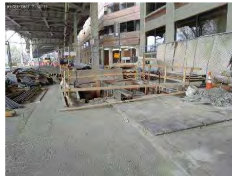
Str 44 Work at Wisconsin Ave
