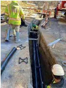
Installing Duct Bank at CSO 029
