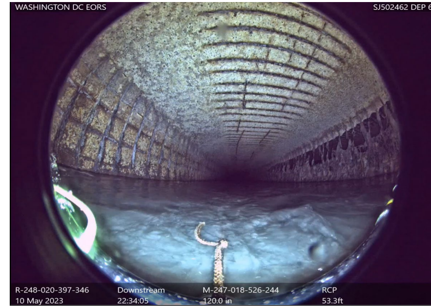
East Outfall Relief Sewer – 50 feet from Structure 2A looking down stream
