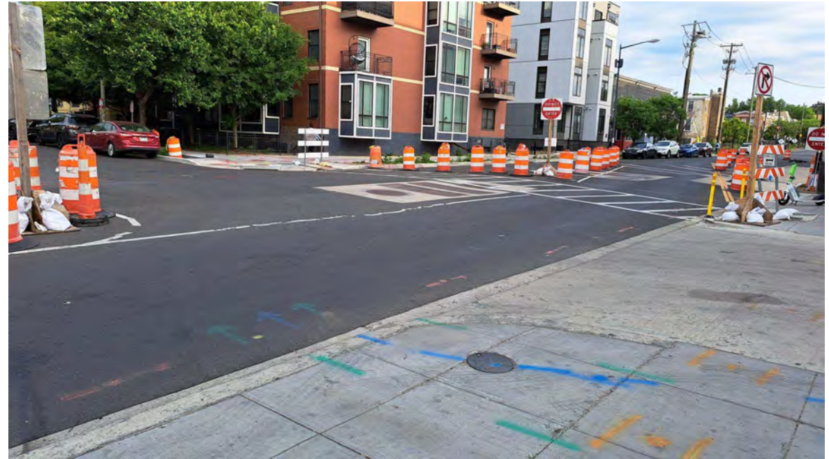
4 th Street Restoration
