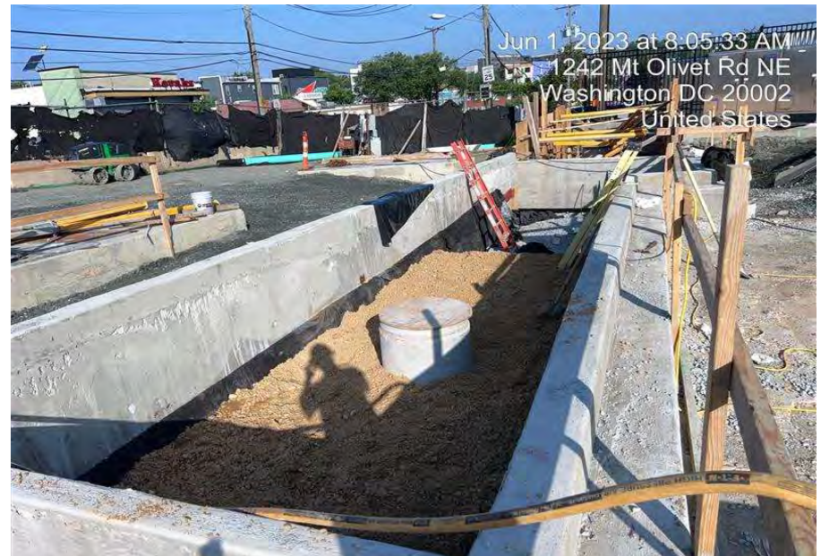
MOR Shaft Bioretention Pond Construction
