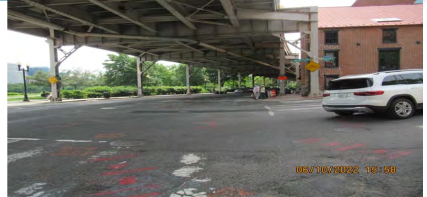
Pavement at the Beginning of Construction
