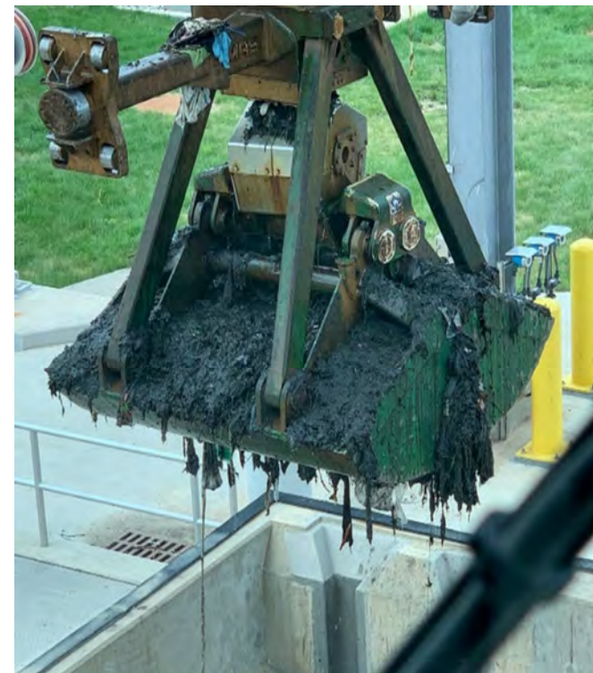
Trash, Debris and Solids Removal from Screening Shaft at Tunnel Dewatering Pumping Station
