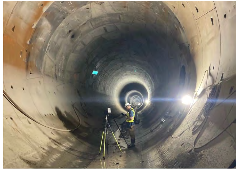
Tunnel Lidar Survey
