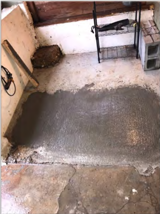
✓ Good Concrete Restoration
