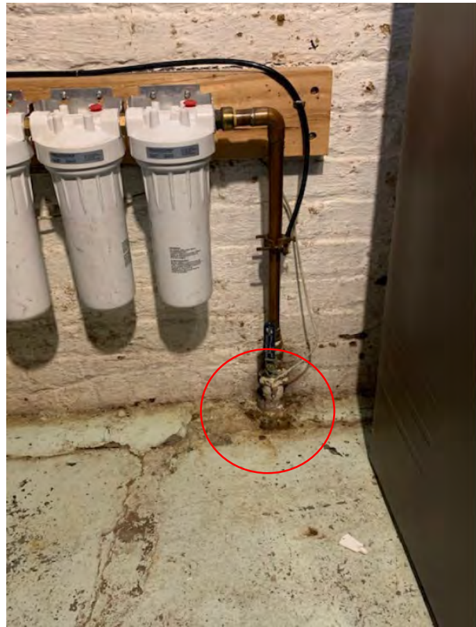
✓ Good 1 st Fitting Pic Breaking through Floor
