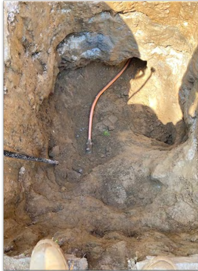
✓ Clear Copper Curb Stop Connection
