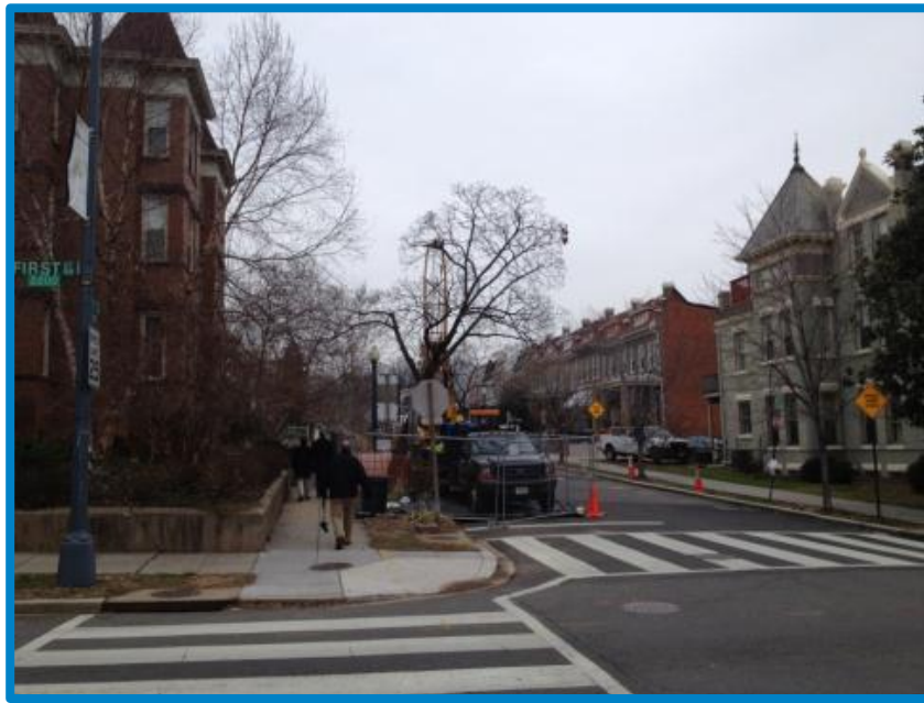
Photo 5-7: Geotechnical Borings Taking Place Along First Street (Photo Taken February 2, 2013)
