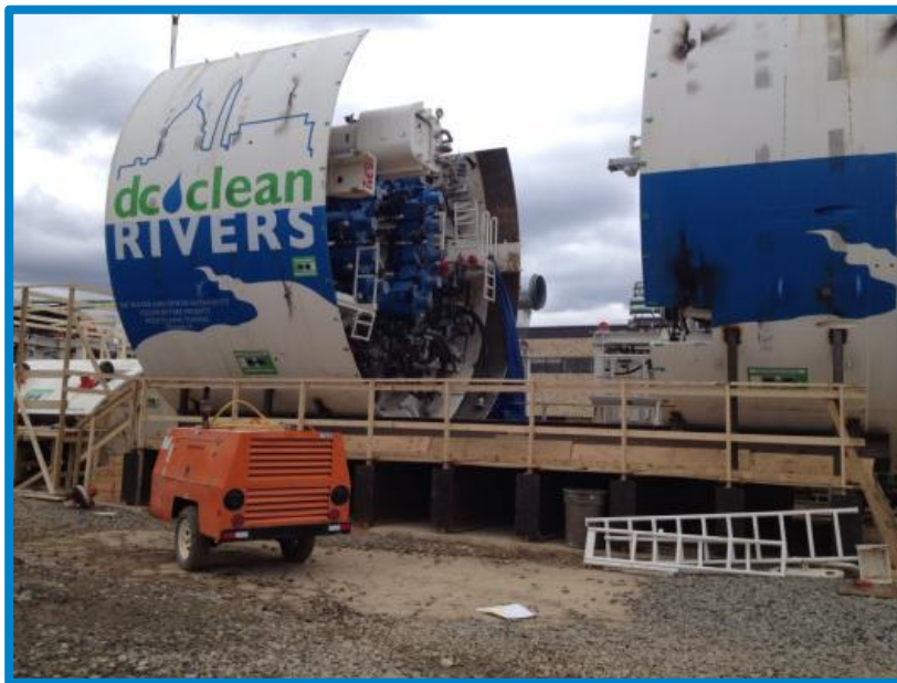
Photo 5-1: Tunnel Boring Machine (TBM) at BPAWTP (Photo Taken March 1, 2013)
