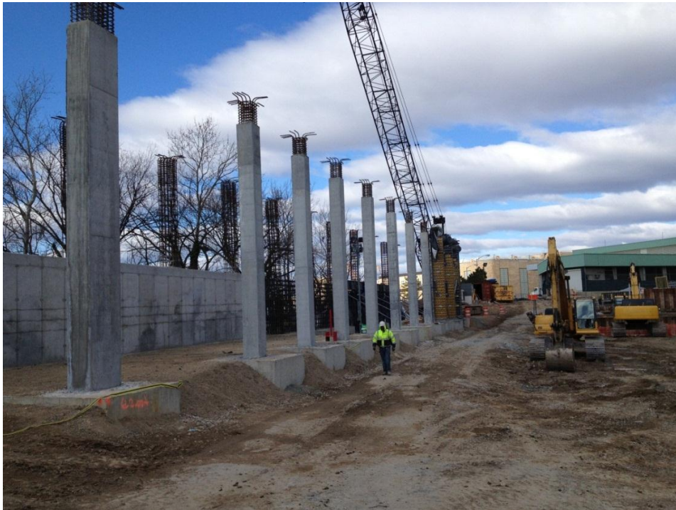
Photo 5 – Belt Press and Truck Loading Facility Under Construction. Photo taken March 8, 2013
