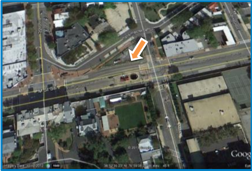
Exhibit 5-12: CSO 015 Under Construction (Image from Google Earth)
