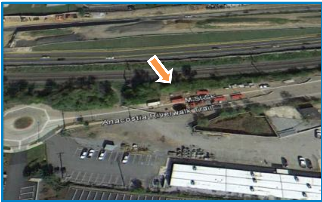
Exhibit 5-13: CSO 017 Under Construction (Image from Google Earth)
