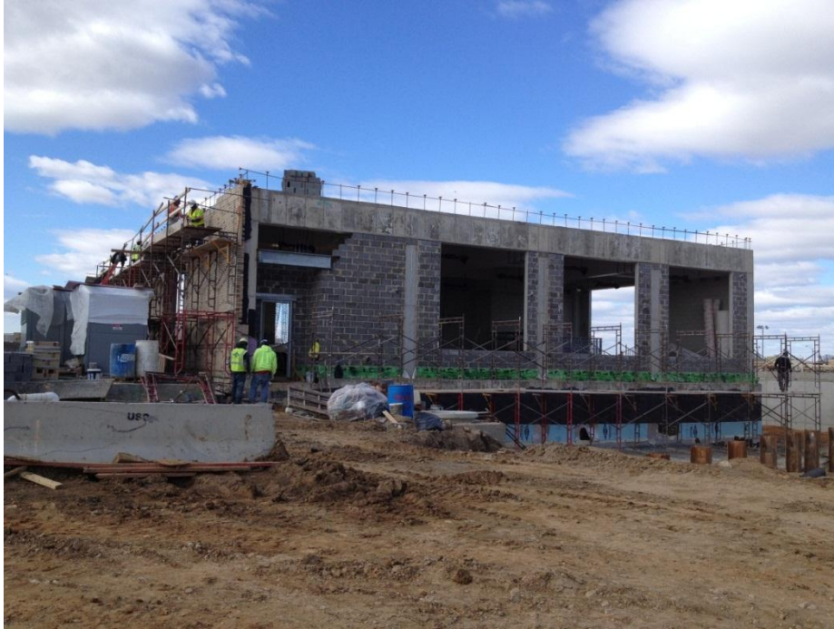
Photo 2 - New Electrical Building for 1 BGD Nitrified Mixed Liquor Pump Station
