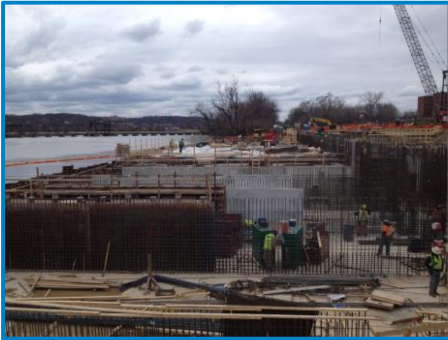
Photo 5-4: Construction of CSO 019 Overflow Structure (Photo Taken March 1, 2013)
