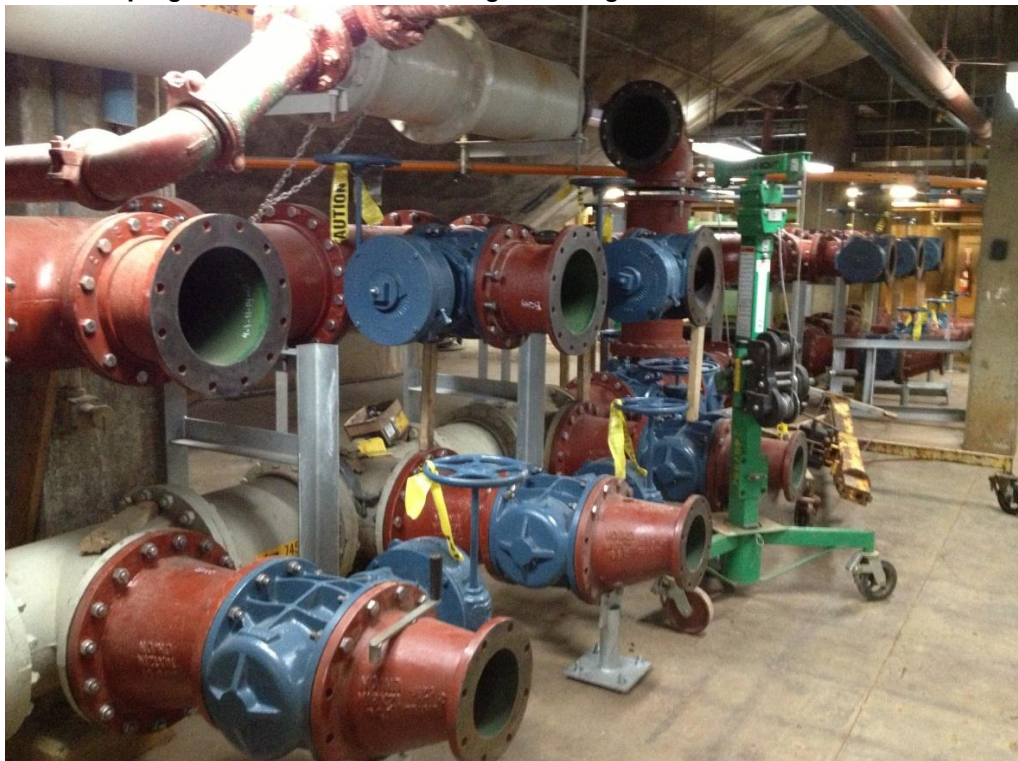
Photo 4 - Piping Modifications to Existing Blending Tanks. Photo Taken March 8, 2013
