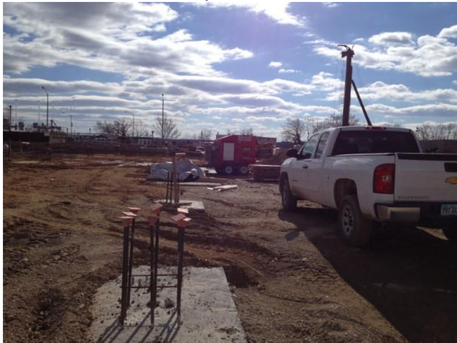
Photo 6 - Central Heat and Power Facility Under Construction. Photo Taken March 8, 2013)
