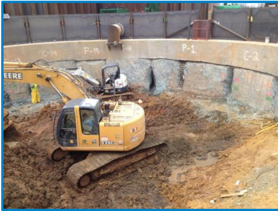
Photo 5-3: Construction on the Poplar Point BPT/ART Shaft (Photo Taken March 1, 2013)
