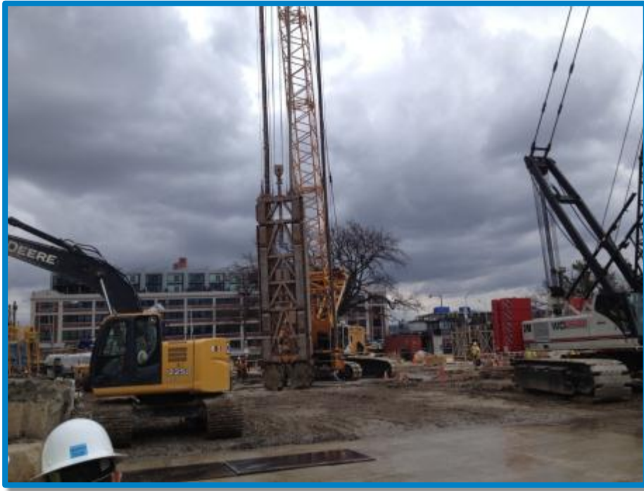
Photo 5-5: Main Pumping Station Drop Shaft Construction (Photo Taken March 1, 2013)
